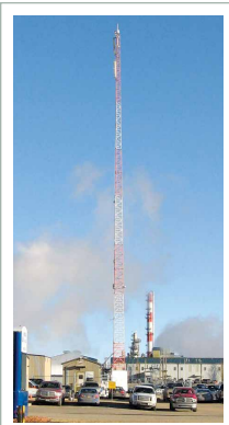
Existing radio tower at the Joffre Site. The proposed new towers are similar in appearance.
