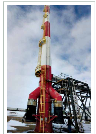
Variable frequency drives were placed on the PE2 flare stack blowers.
